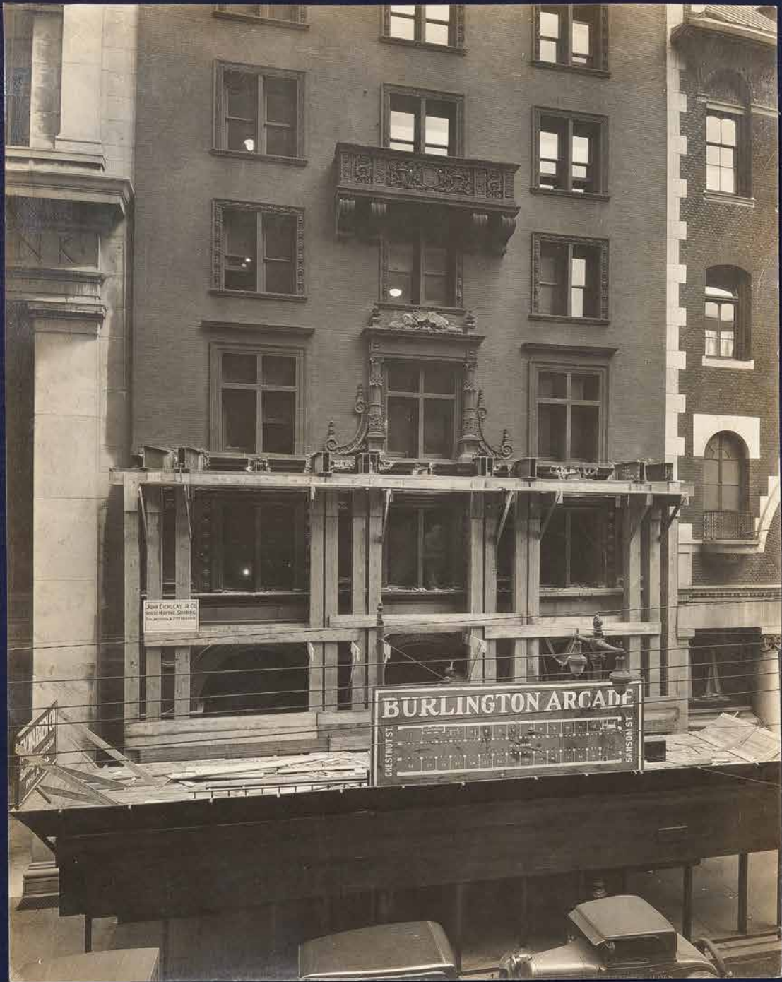
CROZER BUILDING Shoring in place.
