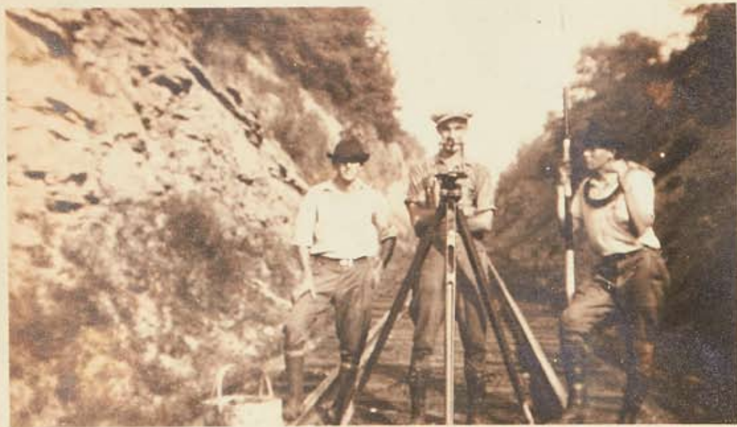
Kensington Cut on Old Main Line— Fox - Dorr Collier
