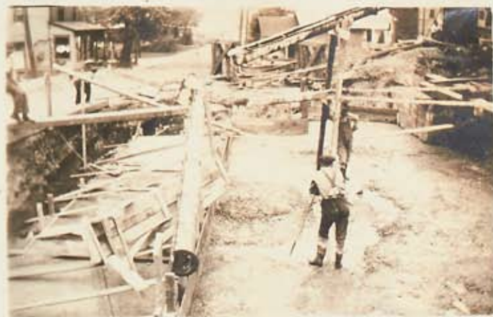
E. Abutment Kens. U.G. Looking North
