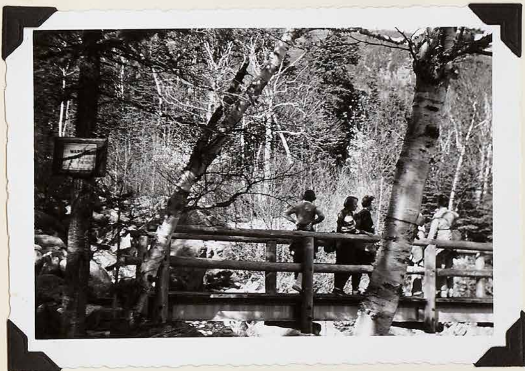
Across the Cutler River on the fire trail in Tuckerman's Ravine
